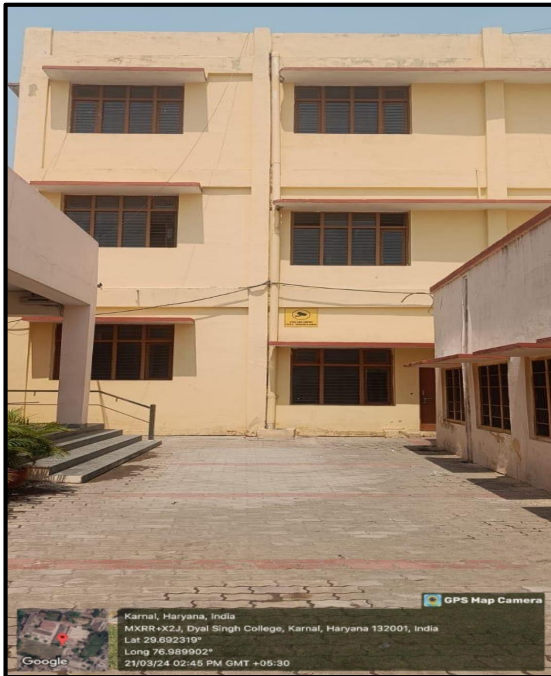
Rain water Harvesting System
