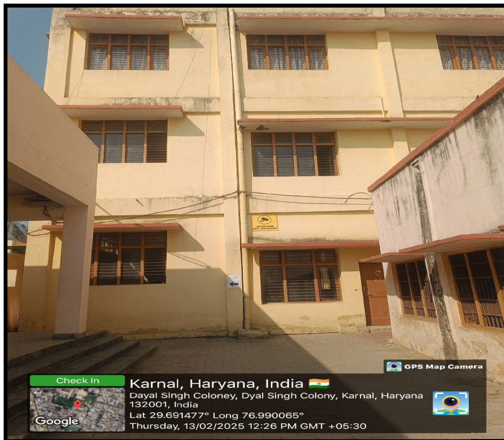
Rainwater Harvesting System
